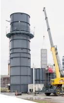
Installation of upgraded silencer panels for FS7F.
