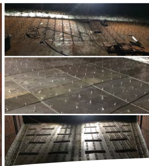
501F duct floor repair.
