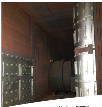
Various FS7EA exhaust liner repairs.
