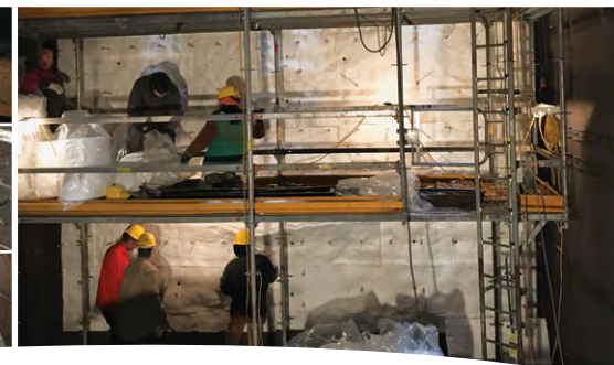
Installing high-temperature insulation on back wall of 7F elbow.
