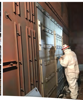
Proper torquing of the exhaust liner hardware.
