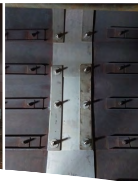
Field relining of exhaust diffuser joint.
