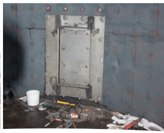
Interior view of universal door frame to accommodate existing stud.
