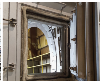
View of high-temperature gasket layers.
