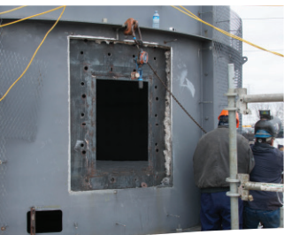
Casing plate prepared for new door frame.
