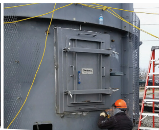
New Schock door in 7F breech duct.
