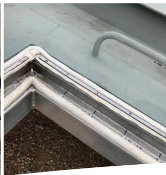
Double gaskets are field-replaceable.
