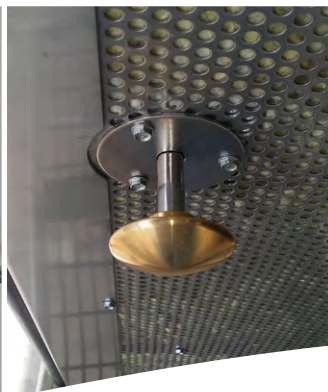
Brass push knob release, with SS stem and mounting plate.
