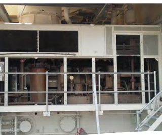
Same site as above, prior to installation of new doors.
